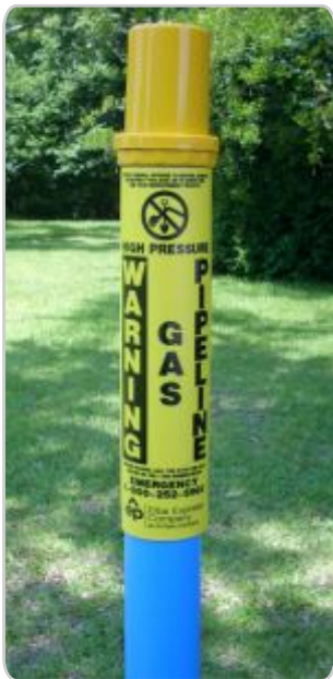
CATHODIC TEST STATION WITH SCREEN PRINTED WARNING MESSAGE
