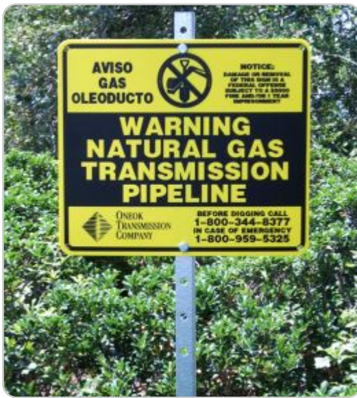
(HDPE) WARNING SIGN ON GALVANIZED ANGLE POST
